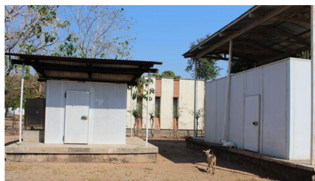
Figure 8: Cold rooms not in use at Nkhotakota District Fisheries Office
